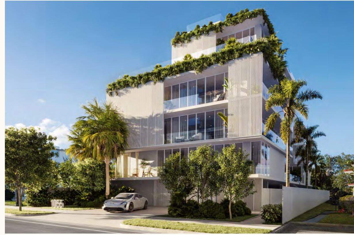
SOLINA Bay Harbor Islands, Miami 22 Condos | March 2023 Completion
